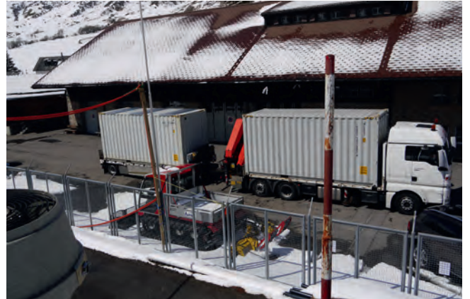
Transport to site Transport zur Baustelle
