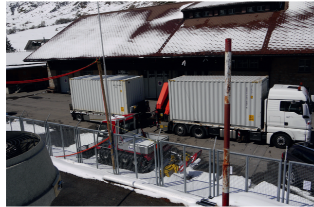
Transport to site Transport zur Baustelle
